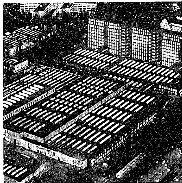
Switchgear Factory in Berlin, Germany
